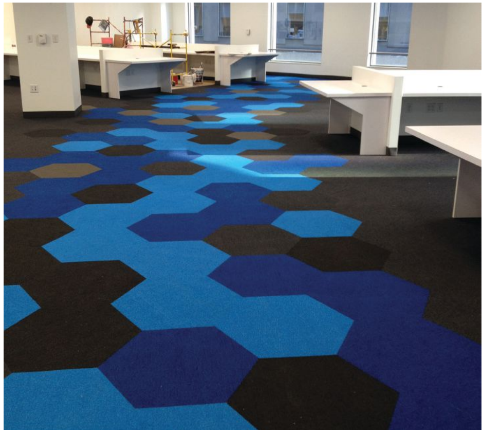
Golden State Carpet Service (GSCS) worked with both the designer and mill rep for the offices of Medrio in San Francisco. This allowed GSCS to communicate to the installers how the designer wanted the hexagon tiles to flow throughout the office. It worked with the designer to approve a mock-up on site prior to installation, as well as collaborated with the designer, end user and installers during installation to make sure the pattern was laid out to meet the client's vision and expectations.
